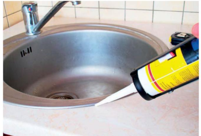
Figure 28.24 Silyl modified polymers (SMPs) are a safer option than traditional adhesives, which use potentially harmful organic solvents.
